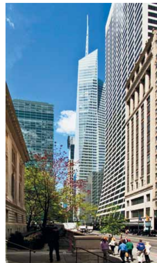
Bank of America Tower, COOKFOX Architects, Нью-Йорк (постройка)
