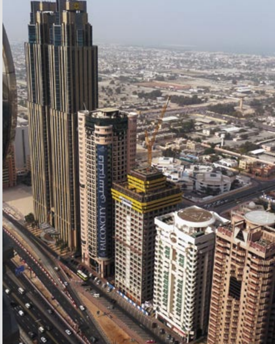
Prime Tower, Дубай
